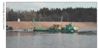
The dredging of the Bay of Örserum started in April 2002. The operation is carried out from a dredger that carefully sucks up the sediment. The slurry is pumped on shore through a buoyant pipe.
